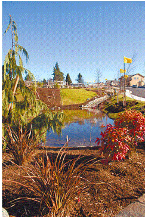
This rain garden is among a number of strategies Shamrock Heights employs to manage stormwater runoff. Homes are clustered to allow space for ponds, swales and natural conveyance.
