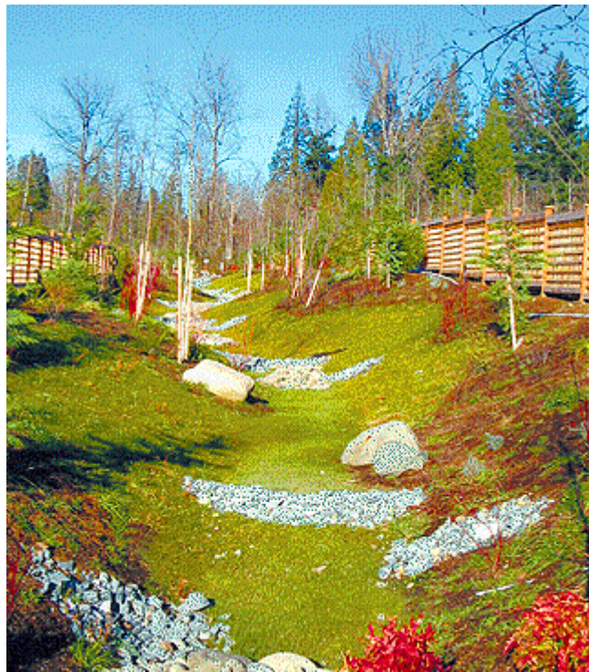
Photos courtesy of CamWest Natural stormwater channels cross through Shamrock Heights, a low-impact neighborhood in Renton developed by CamWest. Wetlands and a greenbelt border two sides. The landscaped channels provide additional open space and buffering between homes.
