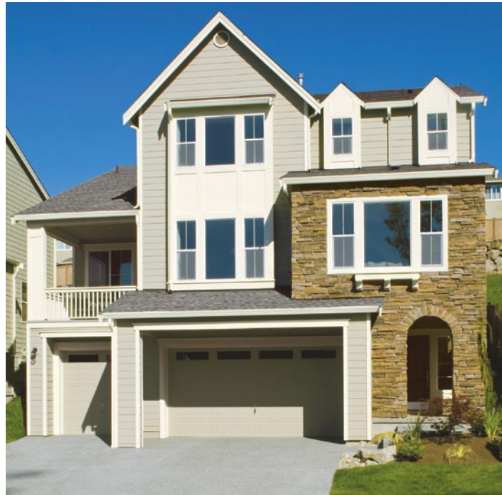
Many of the homes at Cougar Ridge West offer variations on the "two- and three-car garage under" floor plans, which take advantage of the hillside setting.
